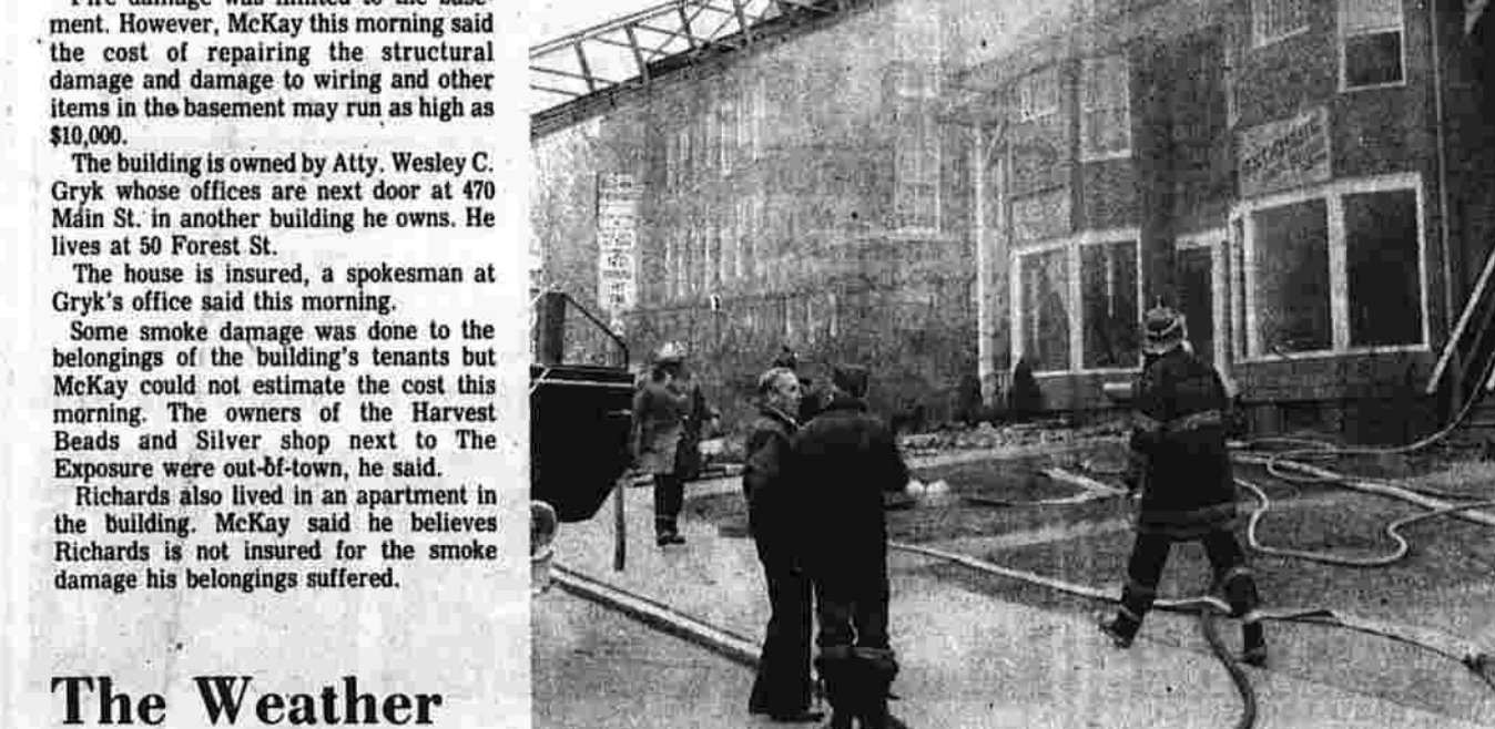
Firemen Rush to Roof
