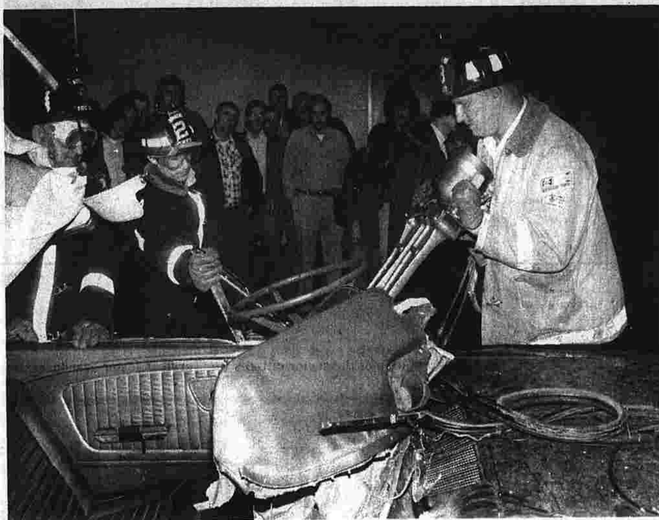
A Hurst rescue tool which tears a car apart in minutes is being demonstrated by Wethersfield Fire Captain William Klatt. The tool eliminates the need for saws and abrasives which also
